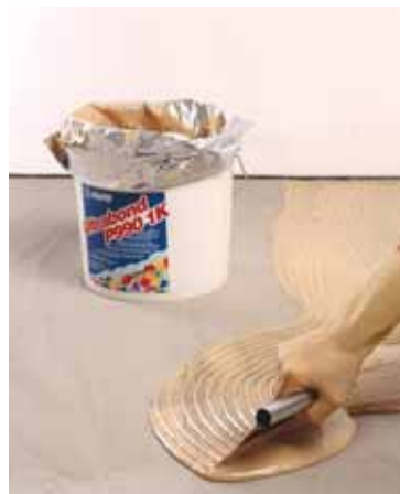
Applying the adhesive
