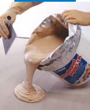
The adhesive is poured onto the screed
