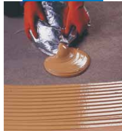
Extracting the adhesive from the interior edge
