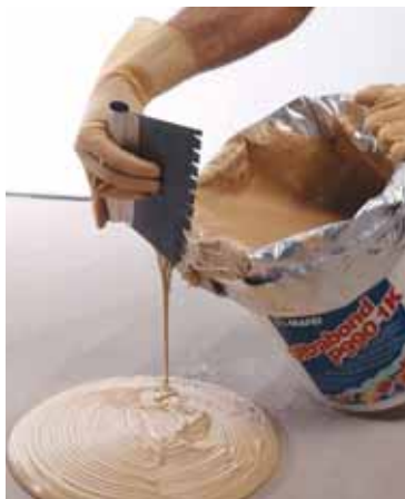
Cleaning off the bucket with a trowel
