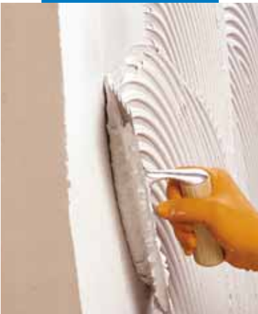
Spreading Tixobond Fine S1 on a substrate
