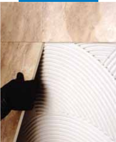
Laying large-sized porcelain tiles on walls
