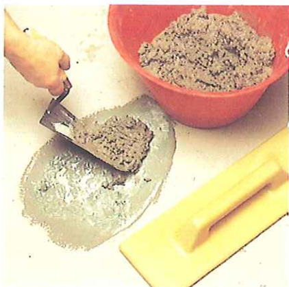
Floor patching: application of mortar
