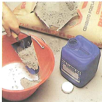
Mixing cement mortar with PLANICRETE SP
