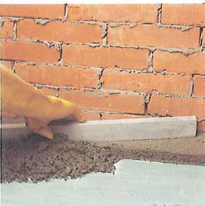
Applying adhesive cement screed modified with PLANICRETE SP
