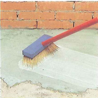
Applying adhesive cement slurry modified with PLANICRETE SP
