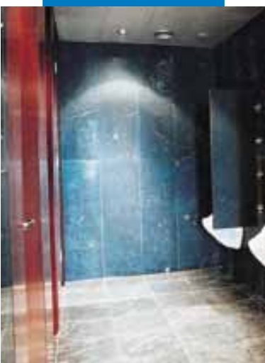
An example of an installation of marble walls with Keraquick - Feuchtwangen casinò bathroom (Germany)
