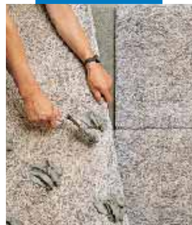
Laying heavy insulation panels
