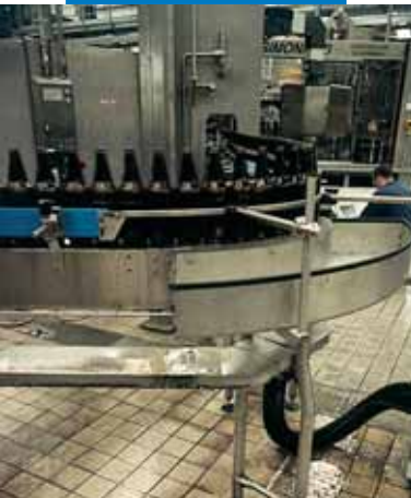
An example of a grouted brewery floor
