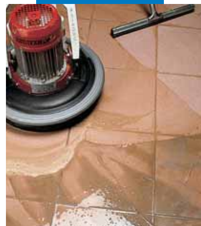
Finishing a porcelain tiled floor with single-brushed power float or rubber rake
