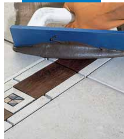
Grouting a ceramic tile floor with wood inlays with a trowel
