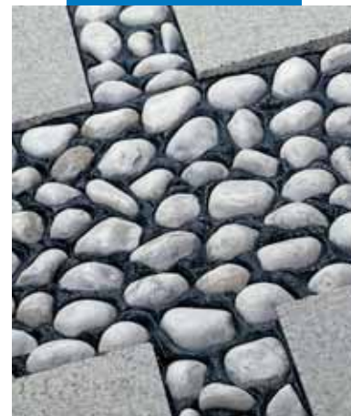
An example of grouted ornamental stones
