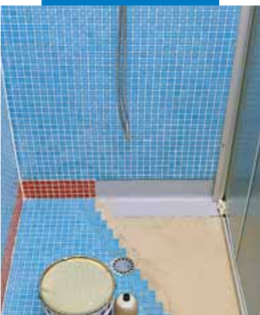
Waterproofing and laying in a prefabricated shower unit
