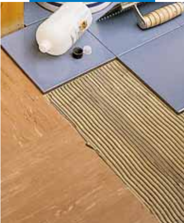
Laying on an old PVC floor
