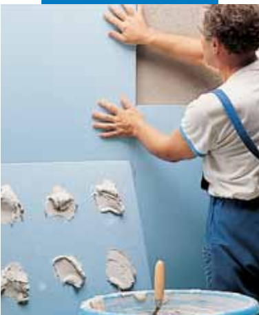
Laying polystyrene foam slabs with Keraflex white
