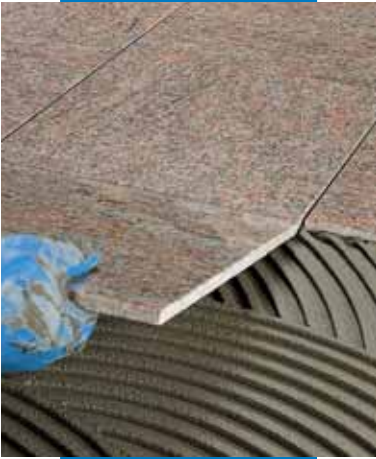
Installation of pre-glossed marble on floors
