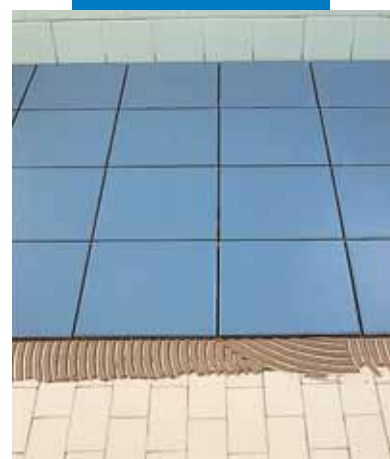
Tile on tile with Keraflex Grey
