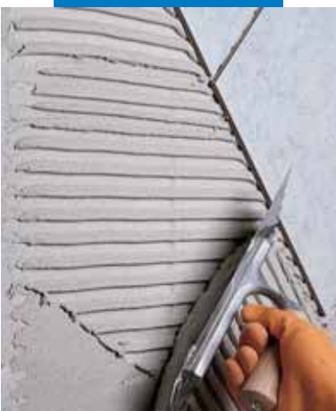
Installation of single-fired tile on expanded foam concrete block walls
